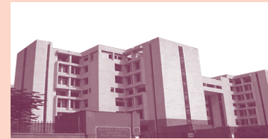
DWARKA COURT COMPLEX p155 - p158
